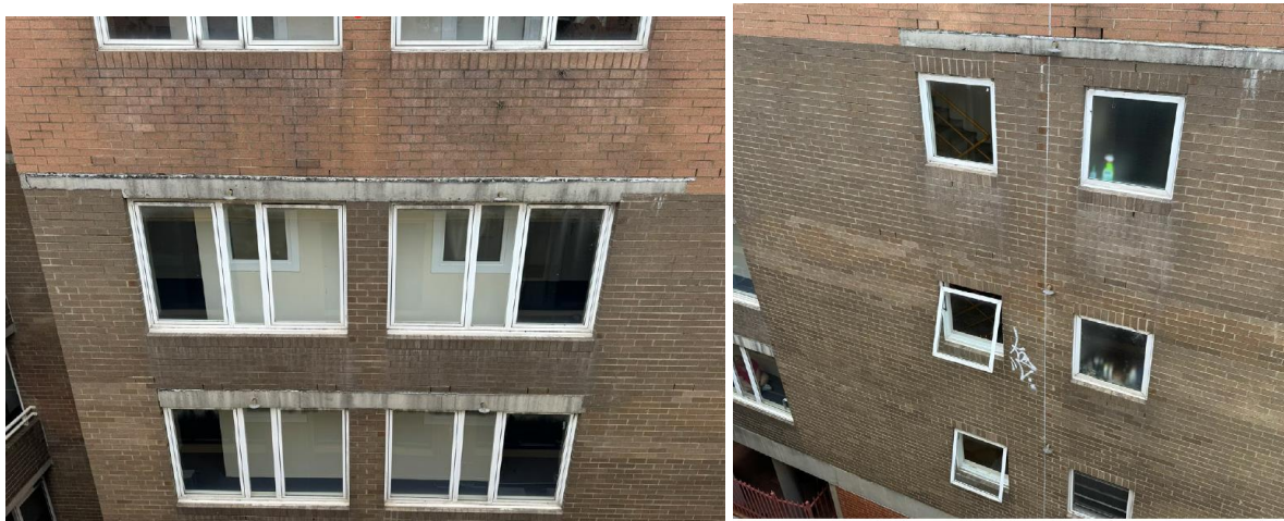
Figure 42: Views to No. 254 Crown Street from subject property showing windows corridors, fire stairs and existing obscured windows
